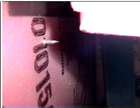
That same nail from the other side. Don't forget to push some spare foam over that tip!
