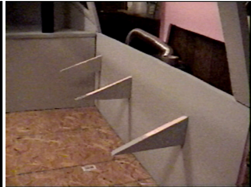
A series of pieces attached to a wall using the dowel method.
